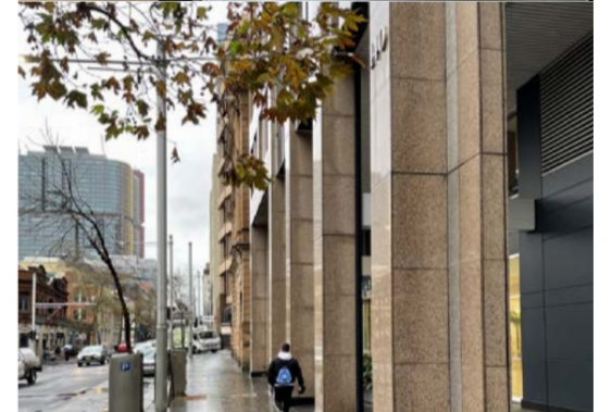
Existing Colonnade at 140 Sussex Street
