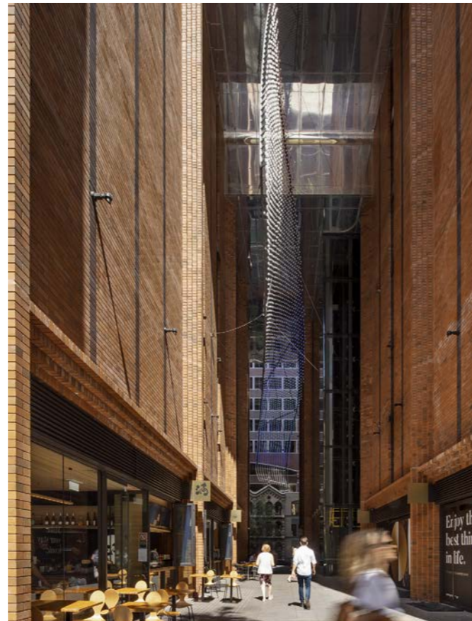
161 Clarence Street - Existing Through Site Link
